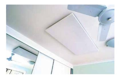
Slimline panels are an efficient and effective radiant heating panel designed to be ceiling mounted. The panels can be used in many applications. The CL750IN has a high IP rating making it suitable for wet areas and outdoor applications.
