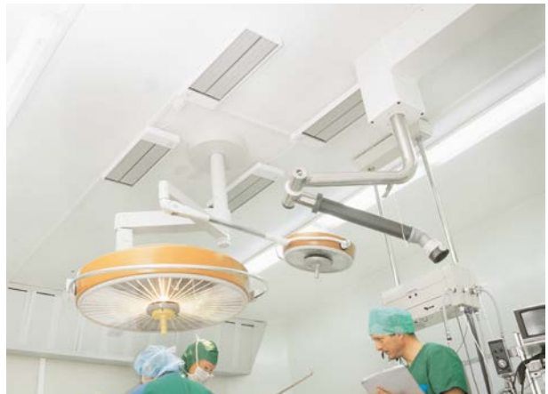
Heating with EZ200 is hygienic since it does not cause any air movements.
