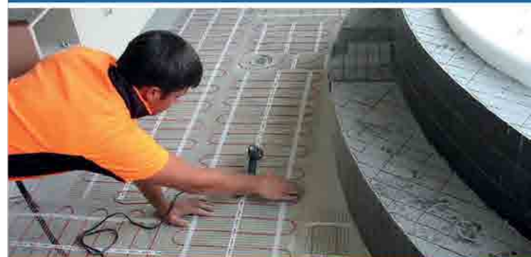
Embedded in Tile Adhesive
